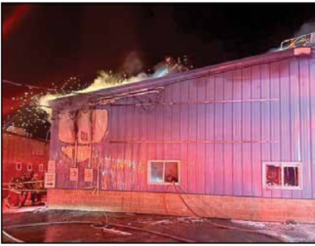
Firefighters responded to 35 Freeport Way in Dorchester on Sunday night around 11 p.m. for a fire in a metal-clad building. The BFD reported one person inside was transported to the hospital with injuries. BFD photo
