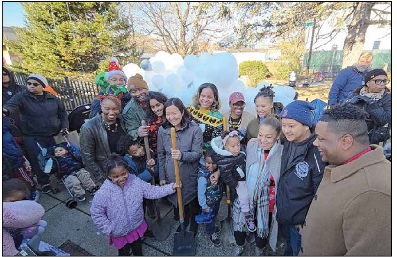
Mayor Wu joined other elected officials and community members in Codman Square on Dec. 1 for the groundbreaking launch of the long-awaited reconstruction of Codman Park, which began on Dec. 9. The park, situated at Washington Street and Talbot Avenue in front of the historic Second Church of Dorchester, is slated to see more accessible walkways and the installation of a stage with electricity for performances and better entry points. Courtesy photo
