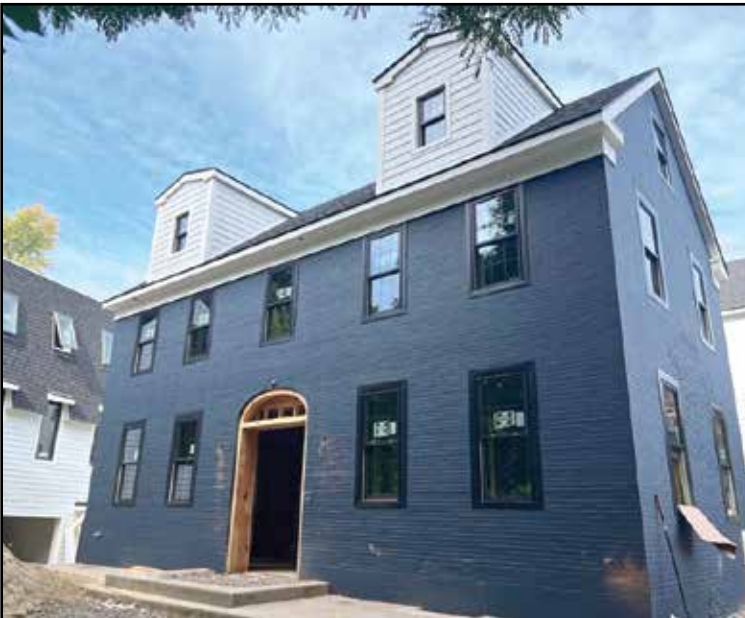
The current state of the Daniel Withington House at 19 Ashland St. in Dorchester. City of Boston image
