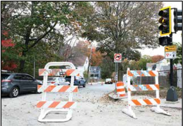
Woodhaven Street has been closed off at Cummins Highway due to the reconstruction there, which has about another year left of work. The situation has left the street inaccessible on both ends.
