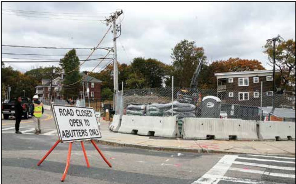
A construction site at 1471 Blue Hill Ave. has closed Woodhaven and Culbert Streets this month, and with the large Cummins Highway reconstruction on the other end of the street – neighbors feel boxed in and ignored.
