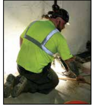
A worker from the lead service line replacement team prepared the lead pipe for removal from a basement in Mattapan’s Standard Street in late August, while guiding in the new copper line that will replace it.
