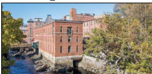
The Baker Chocolate Factory apartment building was sold to Wingate Companies last month for $41 million. The building is located on the Neponset River in Lower Mills. Photo courtesy CBRE
