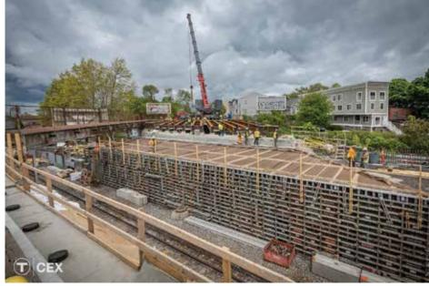
An image supplied by the MBTA shows the erection of structural steel girders on the Dorchester Avenue bridge in May 2024.
