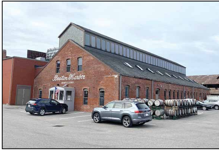
The building at 12R Ericsson St., now housing the Boston Distillery, was termed by the BLC as being a “rare survivor of its type and form.”
