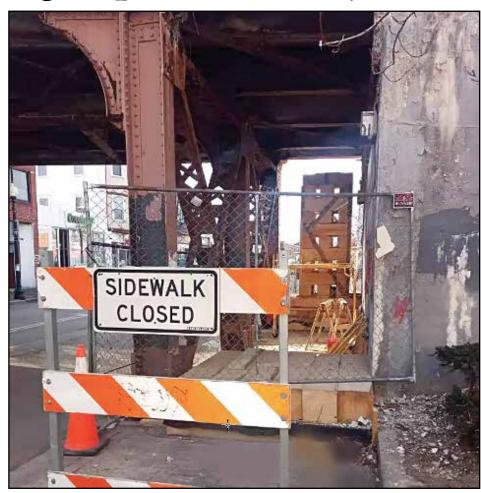
Repair work is underway on this MBTA bridge in Fields Corner to replace concrete and rotten timbers on a walkway.
